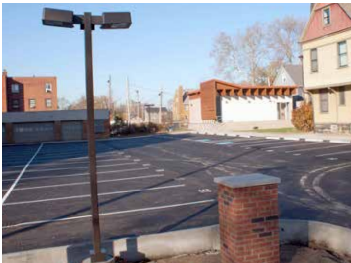
Completed Parking Lot Project. Закінчений Проект Парковки.
